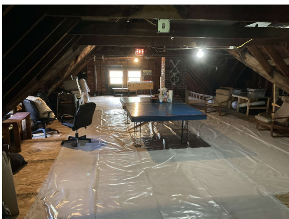
Cleaned out Attic
